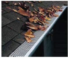
**Type of filter:** (1) In-line; (2) Leaf screens, placed over gutters at the top of the downspout; (3) Diversion by roofwashing with a 4-to-6-inch PVC standpipe (with a valve and bottom cleanout) connected to a gutter downspout. The first rainfall that falls, at a rate of 10 gallons for every 1,000 sq.ft. fills the standpipe, and the rest flows to the downspout connected to the cistern. When the rain stops, the standpipe is drained in preparation for the next rain.
