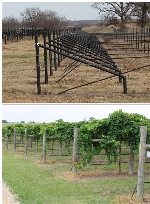
Figure 5. Dead man made from drill stem pipe (top) and H-brace made from wood posts (bottom).
