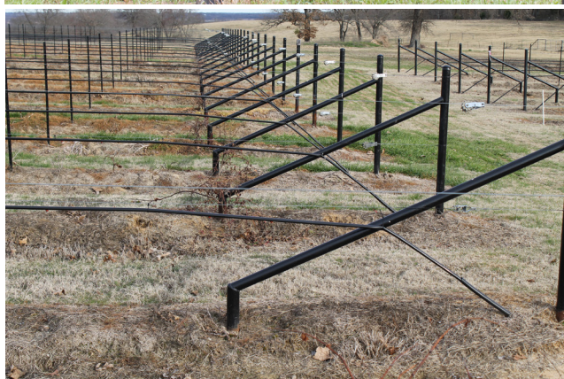
Figure 7. End post assemblies from top to bottom are Tie Back; H-Brace; and Dead man.
