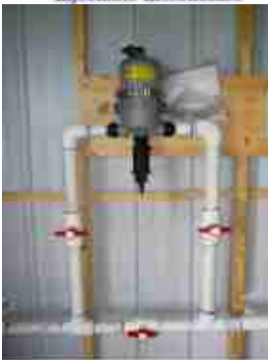
In the "Closed Position", Mechanical Injection Pumps Can Simplify Accurate Injection Through Drip Systems
