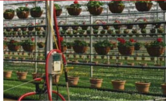
Installation of flow meters in each bay, section or greenhouse allows for crop-by-crop assessment, and the assessment of individual growers if this applies.
